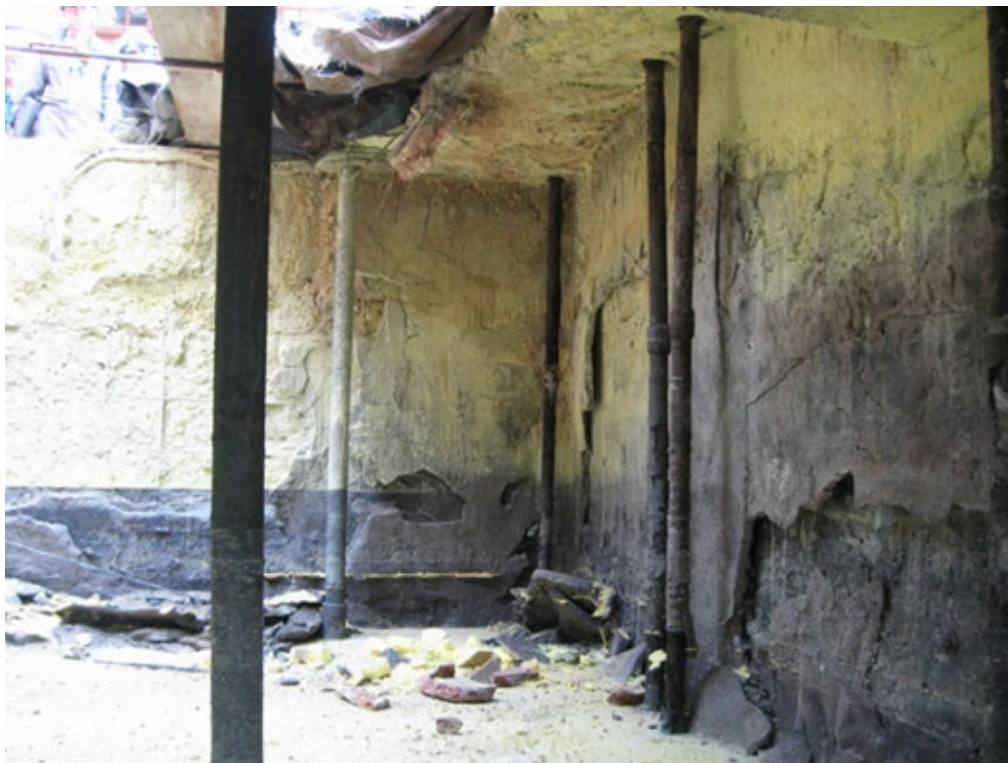
Figure 1: Sulfur pit roof and wall failure due to lack of maintenance bringing down Sulfur containment in a Sulfur Recovery Unit at a Southwest USA Petroleum Refinery.
